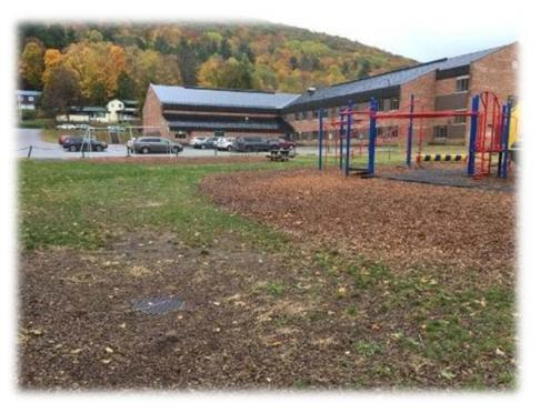
Figure 4: School 001 (northern) site. The inlet to the existing dry well is shown in the foreground. The system of chambers would be installed underground directly off the edge of the parking lot's paved area.
